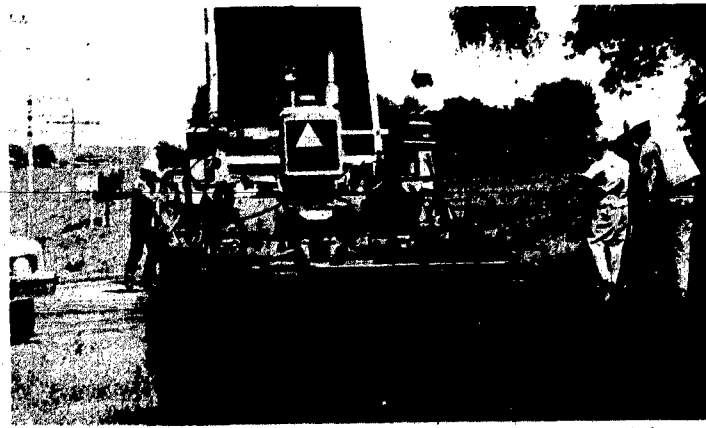
WORK STARTED last week on Highway 15 just south of Laurel. The $183,000 project may be completed in eight working days.
